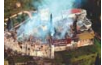
Chilantari durante el incendio. Chilantari during fire.
